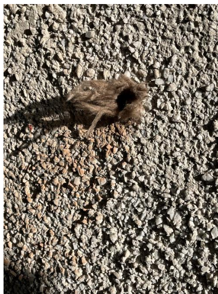
Exterior Wall Insulation
