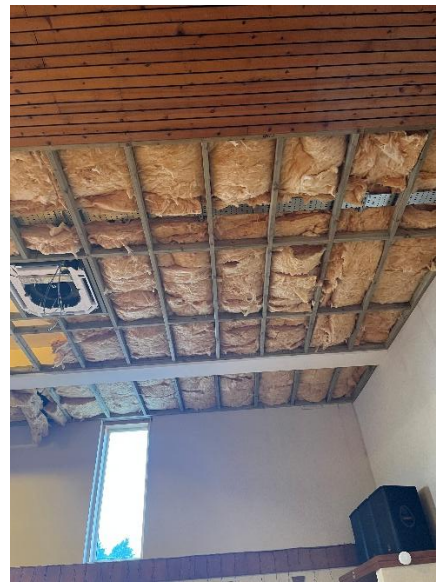
Void Filling in Ceiling - After
