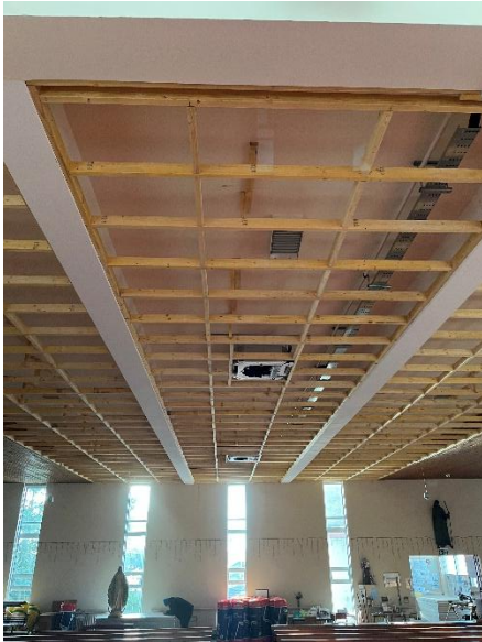
Void Filling in Ceiling – Before
